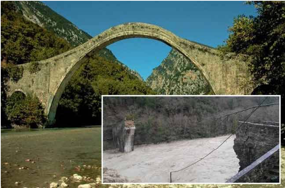
Image of the historical Plaka Bridge, before and after the collapse on 1 FEBRUARY 2015.
